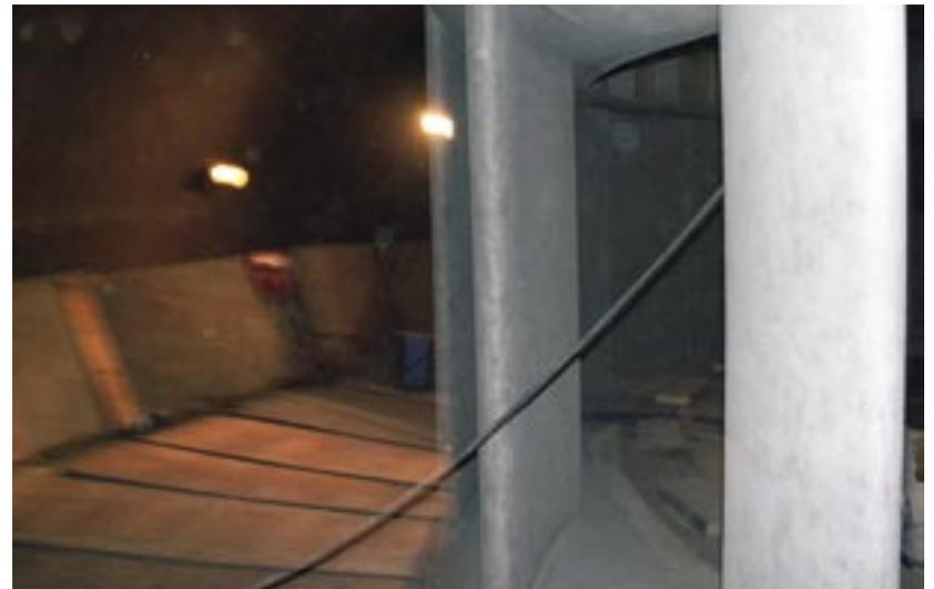
*The new Sponge-Jet method was used for the first time in hydro electrical power plants such as Stornorrfor, which is Sweden's second largest power plant. The guide rails and bar columns were blasted, saving the power plant nearly €84000.*
