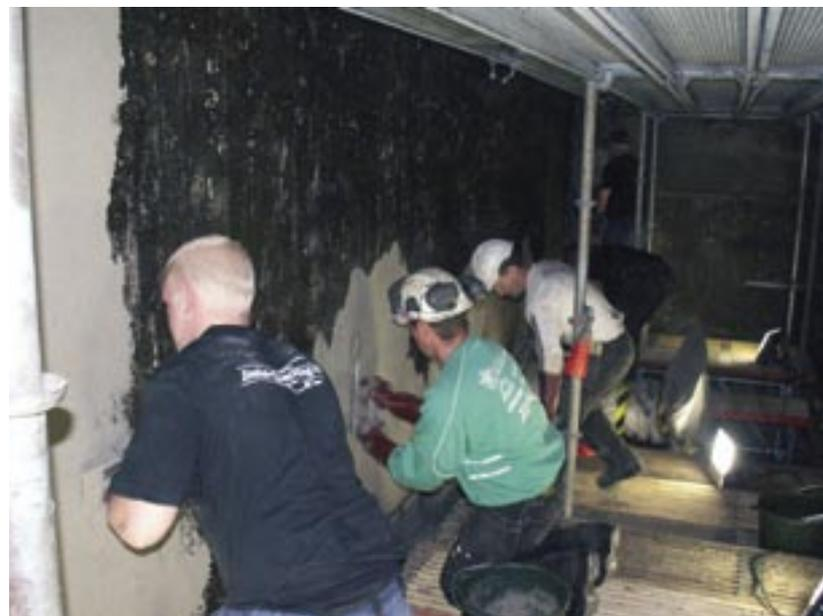
Over five days the walls in the stock chest should be rebuilt with fast curing cement based repair material and then coated with composites.
