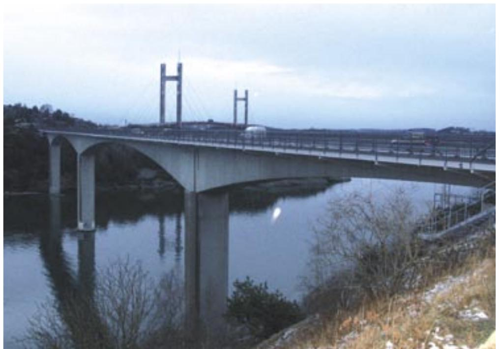
One of the two bridges that joins the island Tjörn with the mainland on the Swedish west coast has been strengthened with carbon fibre composite.
