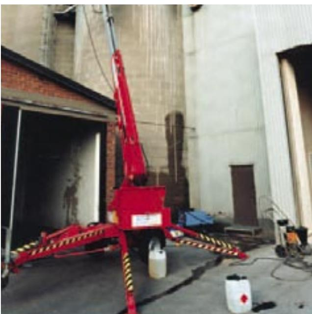
Silos, chimneys, water towers, walkways and other buildings/constructions carbonate because of weather, acid rain, chlorides, etcetera. It is important to protect the assets by cleaning, repairing and shielding in time, before much larger and more costly repairs have to be carried out.
